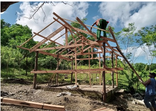
Restoration of Endemic Tree Nursery (ETN) House
